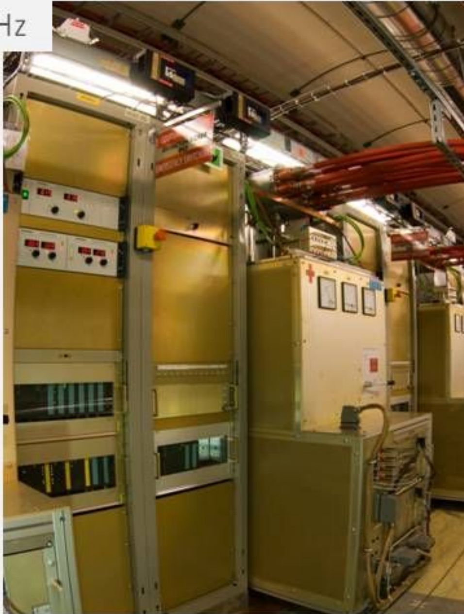
Fail-safe SIEMENS SIMATIC S7-F Programmable Logic Controllers
