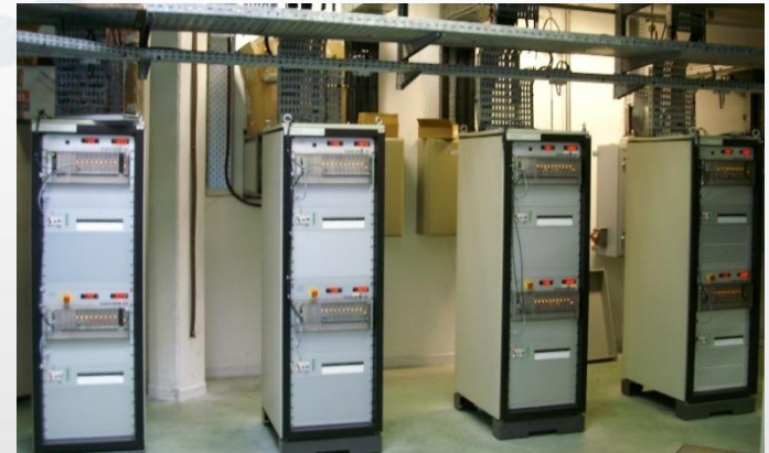
1/4 of the steerers DC Power Converters to be replaced by AC-DC Power Converters
